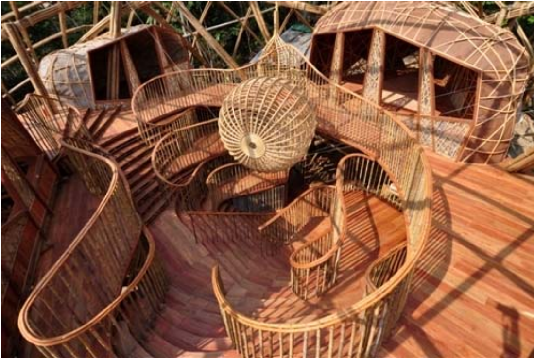
Interior under construction
