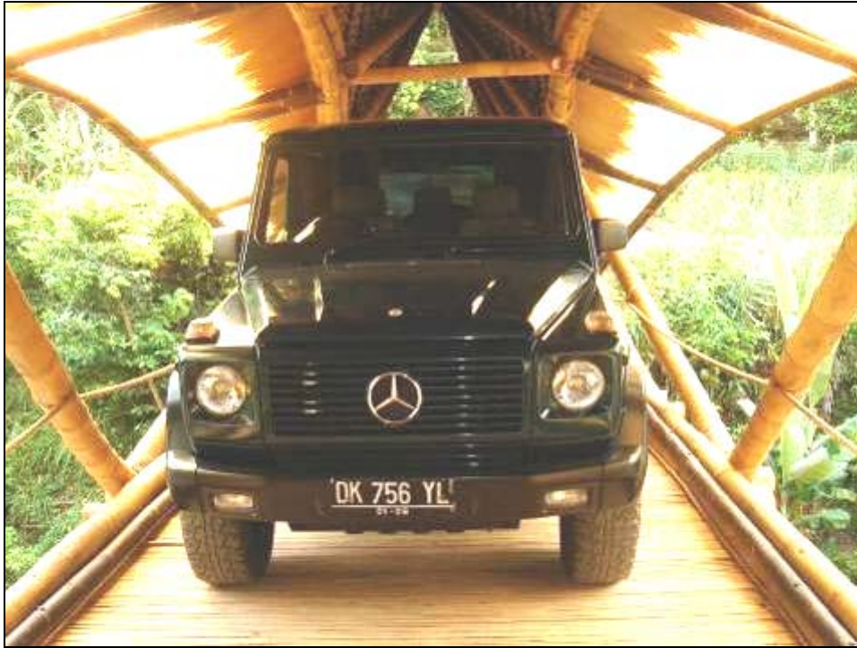
Photo 16: The two arches are composed by 3 bamboos of Dendrocalamus asper , interconnected by steel bolts and bamboo dowels. The floor is made from the cracked poles, using bamboo dowels to join about 20 splits each into glue free Bamboo board, called “PinBoo”.
