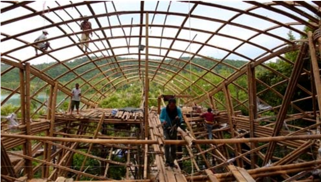
Roof structure under construction
