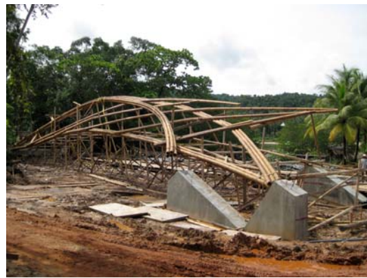
Left- Team Koh Kood, Thailand. Right- Giant truss lying damaged on scaffolding after a failed lifting attempt. Photo shows Primary Double footings, and distorted arch's after damage.
