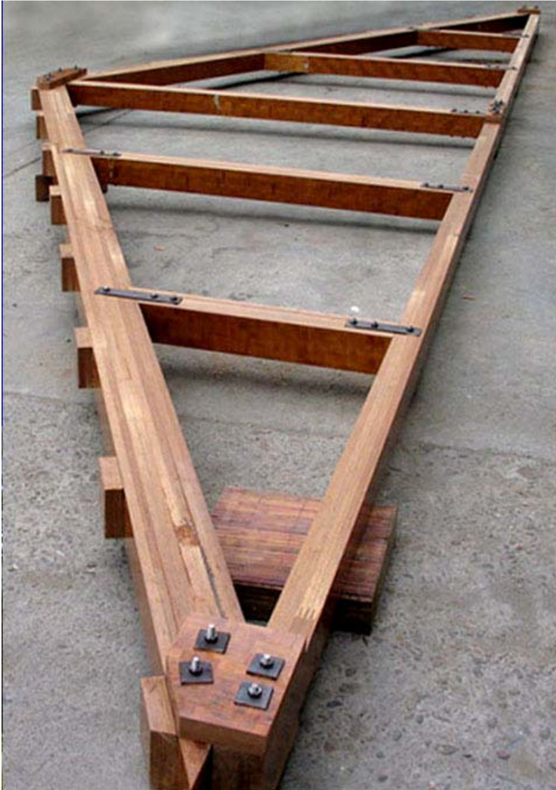
Figure 20 Glued laminated bamboo as roof frame (Courtesy of Chen Xiaon)
