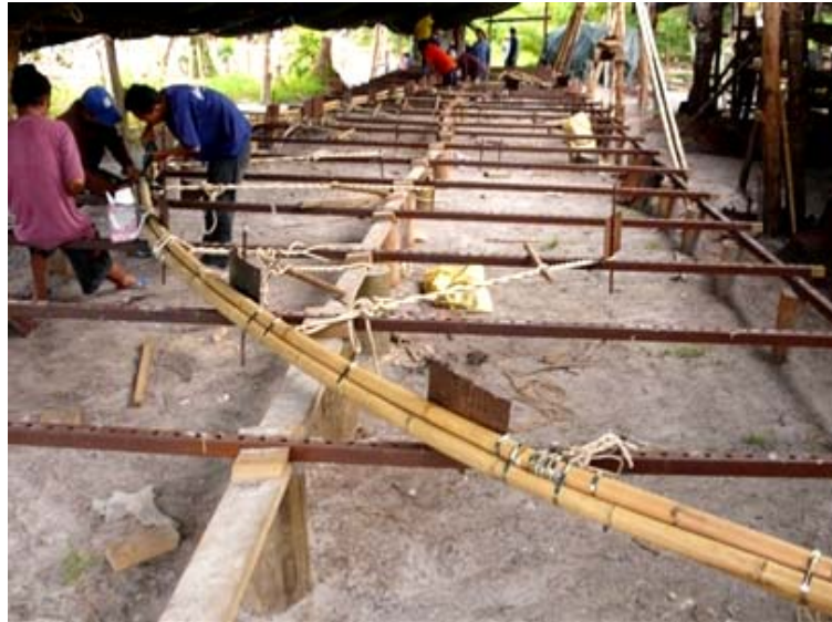
Adjustable formwork for making the curved beams
