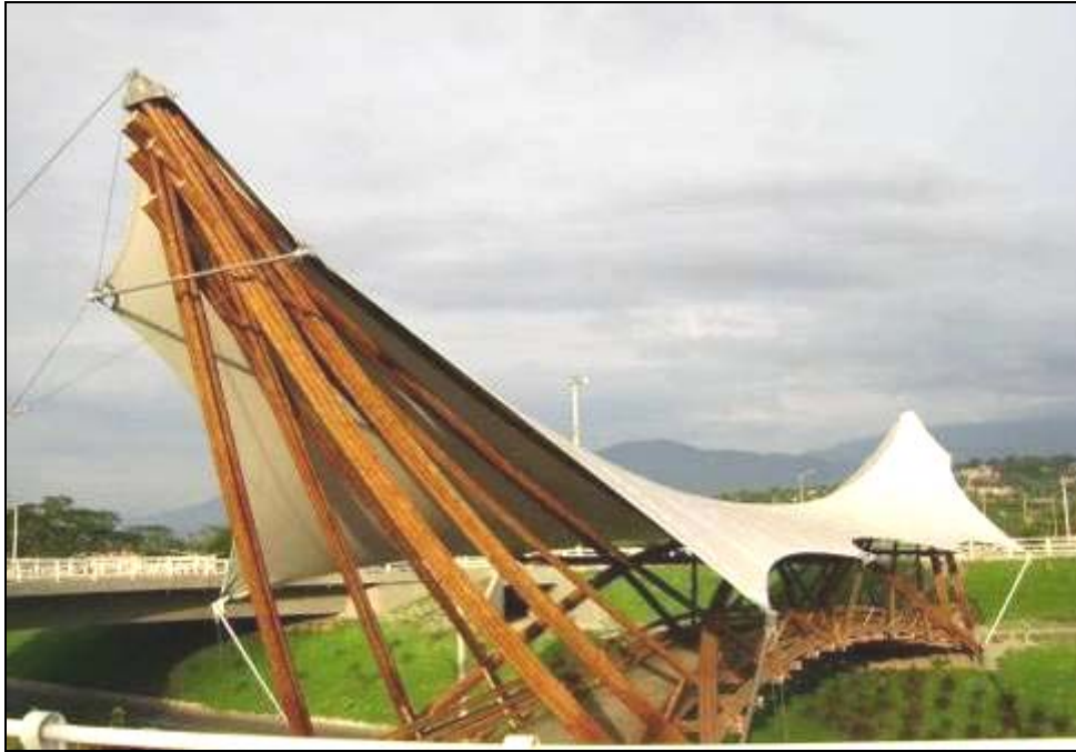
Photo 13: The 400 m 2 membrane allows sufficient weather protection for the bamboo poles. Its cables are actively involved in strengthening the tower and help to support even the floor beam at the center. Although on the photo the morning sun still hits the tower, but the bridge is quite protected by the membrane at noon. The bamboo is painted with an open poring natural oil firnis, which includes UV protection and antifungal agents.
