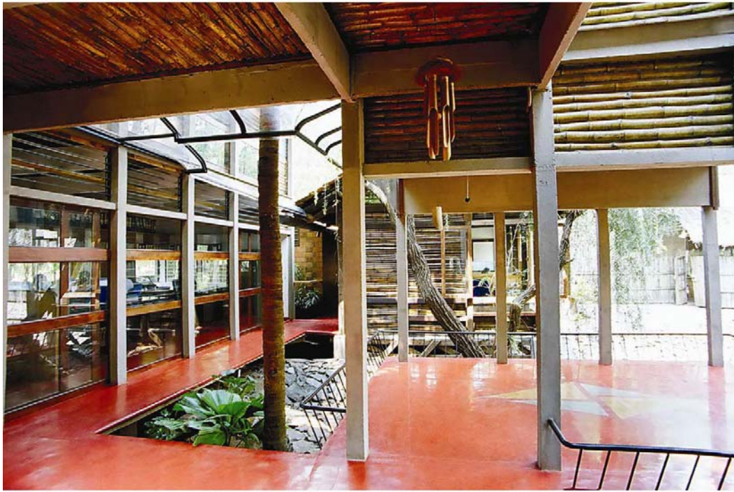
Figure 3 – Inspiration Office: Exterior Front View ; Bamboo-reinforced Mortar Floor Slab finished with Polished Red Oxide
