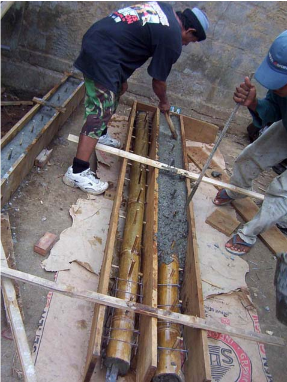
Figure 22 Utilization of bamboo pole as reinforcement for prefabricated concrete beam
