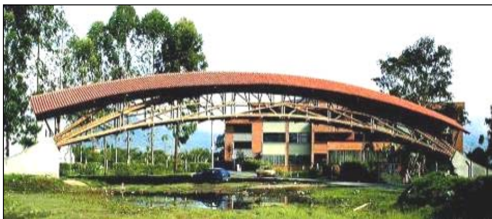
Photo 7: The Bamboo Bridge at the technical University in Pereira (UTP) was built during a one month workshop in the year 2000. The 40 meter bamboo arch stretches over a 4 lane road and has to respect a 5 meter clearance. The load test was done in a moderate progression until reaching 250kg/m 2 . The arch flexed only 4 cm, recovered 3,8cm, and is stable since then. The permanent deformation of 2mm is caused by the squeezed fibers at the contact zones with each other and with the thread of the steel bolts. The bridge also survived a lateral impact of a drunken truck driver that forgot to close his “bucket”.
