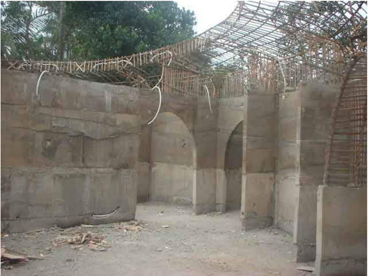
Figure 21 Bamboo split as concrete reinforcement in Bali, Indonesia
