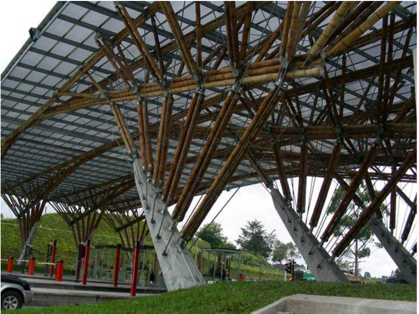
Figure 17 Bamboo as compression element in combination with steel tension wire
