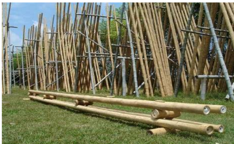
Photo 1: Four guaduas of 8 meters are joined as a “spaced column”.
