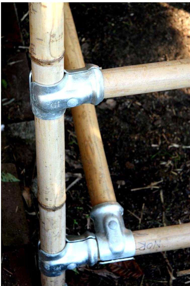
Figure 6 – Connection detail for Chicken Shed
