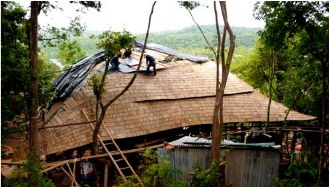
Bamboo shingle roof being installed
