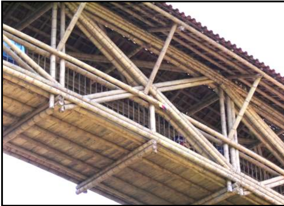
Photo 20: The HOWE concept is a sandwich framework. The tension and compression beams mutually stabilize at the cross over in the center, where usually the worst for buckling occurs. The tension element in the middle layer is bolted in between the outer and inner layer to transfer the forces evenly. The compression beams are cut one-third into the arches and grouted to avoid squeezing. Observe how the traverses are hanging below the floor arch and how the rails under the floor form a “lost casing” with the crushed bamboo mats.
