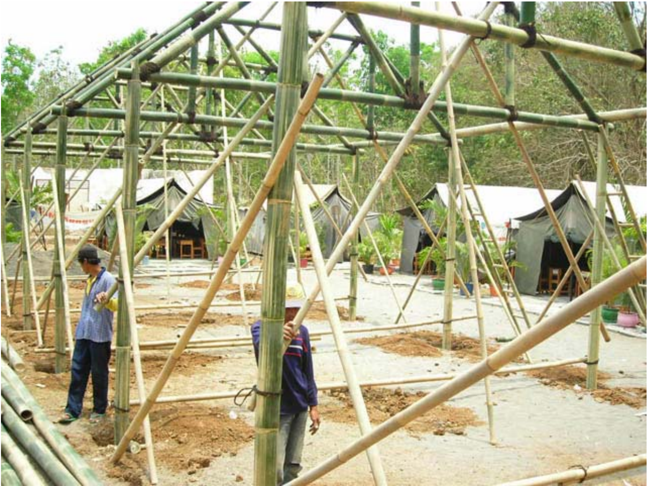
Figure 6 Planar frame in common traditional bamboo constructions (Courtesy of AMURT)
