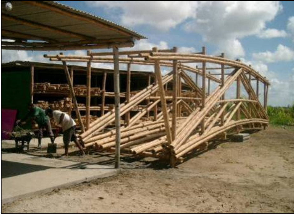
Photo 17: Bridge in form of a “Box”. The KING Truss of 12 meters was made in Guadua chacoensis en Maceio, Brazil. The style is a true copy of successful systems used in the middle ages and colonial times. Traverses double beams are hanging under the floor, which gives more internal height for the passenger. The crushed bamboo mat called “esterilla” provides the formwork, and the floor belt of the truss confines the limits of the concrete slab, which besides having good abrasive behaviour, also stabilizes against lateral buckling.
