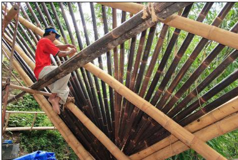
Photo 14: The two opposing directions are shown in yellow ( Dendrocalamus asper ) and in black bamboo ( Gigantochloa atroviolecia ).
