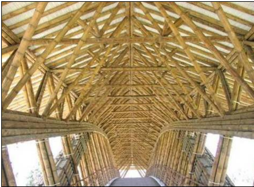
Photo 8: Bridge “Jenny Garzón”, Bogota 2003, designed by Simon Velez and named after the engineer who investigated the grouted bamboo joints for the ZERI pavilion in Hannover. The bridge has a 46 meter span and shows clearly the arch concept and its suspended floor level.
