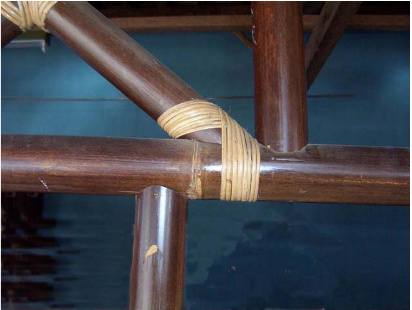
Figure 8 Eccentricity in traditional bamboo connection and the effort to place the connection near to the node
