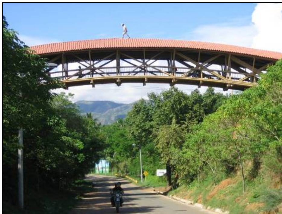
Photo 19: This 30 meter bridge in Santa Fe de Antioquia, Colombia was pre assembled completely on a lawn besides the road. The bamboo structure had a weight of 8 tons and a mobile crane simply lifted it onto the bridgeheads. The entire operation only required a two hour road block and the entire bridge project has being finished in one month.
