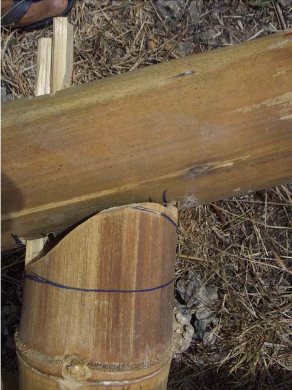
Figure 3 Fish-mouth joint with two pinned flanges (Courtesy of Benjamin Brown)
