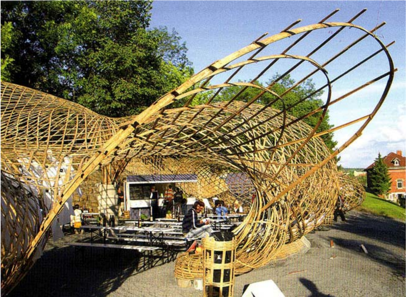
Figure 15 An innovative form made of bamboo split (Kalberer 2007)
