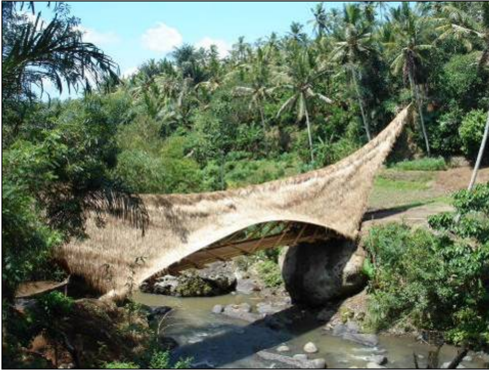
Photo 15: The 22 meter Bridge at “Greenschool” in Sibang, Bali, Indonesia. The two horns are typical ethnic architecture of the Minang Kerbau people from Sumatra and very good for natural air conditioning. The structural concept of the form active surface relies on 4 stiff screens leaning into each other, so the two horns do not require cables to assume the tension of the diagonals.
