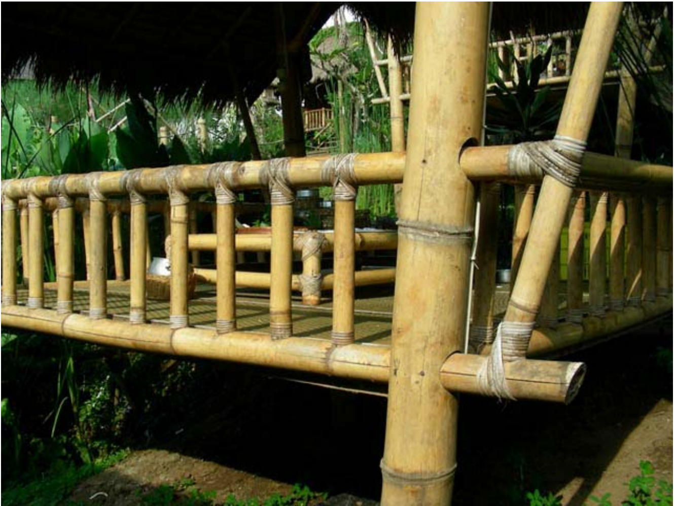
Figure 5 Traditional bamboo gazebo in Indonesia with positive fitting and rope connection
