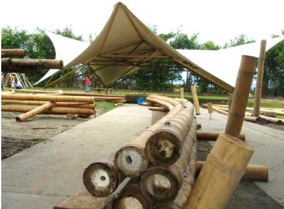
Photo 5: Six curved lines of guadua bamboos are joined to a 12 meter composed beam. The 60 cm pitch is quite powerful, but it will cause a strong reaction in the bridgeheads. The lateral buckling will be controlled by a concrete slab. The connection of the beams with the footing is done with an articulated galvanized steel plate, that allows a reliable fixing on concrete.
