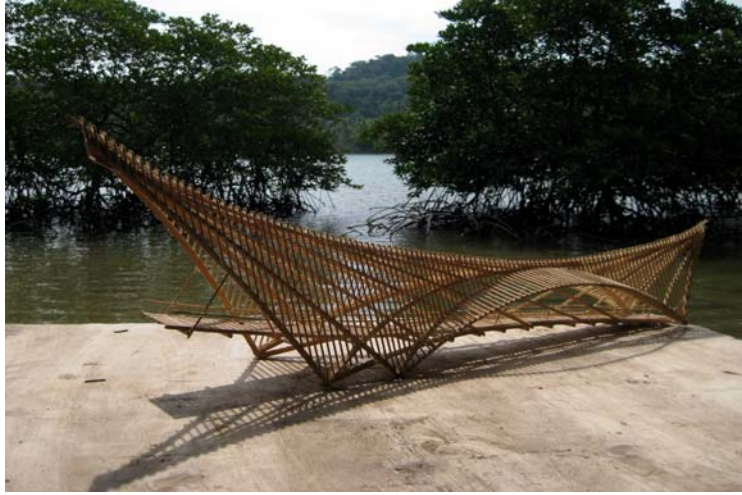
Above- Bridge Cúcuta, Colombia with membrane tarp protecting a symmetrical structure. Below- Model of Bridge at Koh Kood, Thailand currently under construction, to be completed in June 2009. Asymmetrical bridge design with the tension elements radiating from the double footing, whilst at the other end, these apparently similar elements only support the roof structure.
