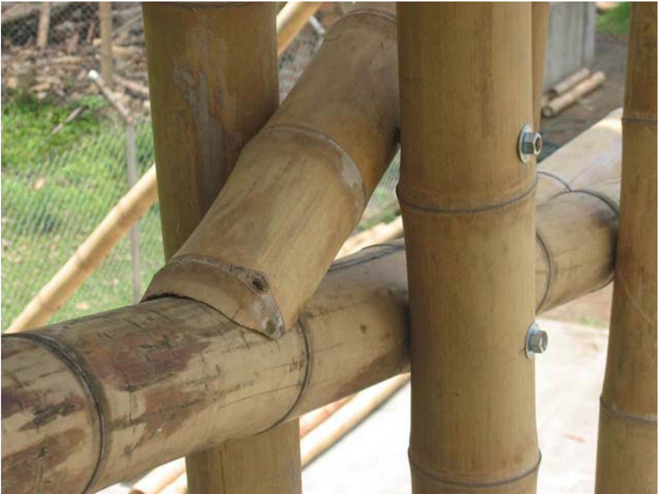
Figure 14 Eccentricity of load transfer in a connection (Courtesy of Jörg Stamm)
