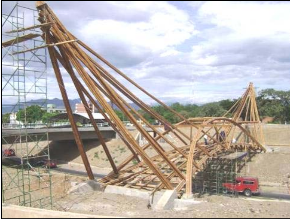
Photo 12: The arch is composed by 6 lines of guadua, stabilized by tension beams. The first “Cables” are actually columns under compression, forming a pyramidal tower, which in reality has to respond more to the loads from the membrane, than from the floor. Most of the bridge load is assumed by the arches, - according to the computer model the tension beams are actually mainly decorative.
