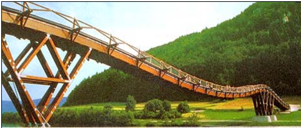
Photo 10: Belt Bridge at the bicycle trail along the Rhine-Donau Canal at the Altmühl, valley in Germany. An about 190 meters long Belt of laminated pine follows the curve of the changing momentum, while it is supported by two towers. The road is the roof which ensures protection by design over the 6 beams of 20 x 60 cm cross-section. The overall length of 190 meters had been delivered in three sections which were glued together in situ with finger joints.
