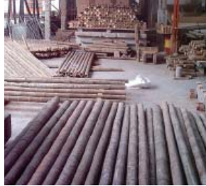
Figure 2. Elements selected and cut for construction of the standard frame
