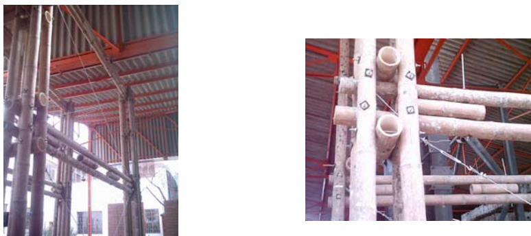
Figure 8. Frame of guadua with diagonal cables. Diagonal cable leaving the joint
