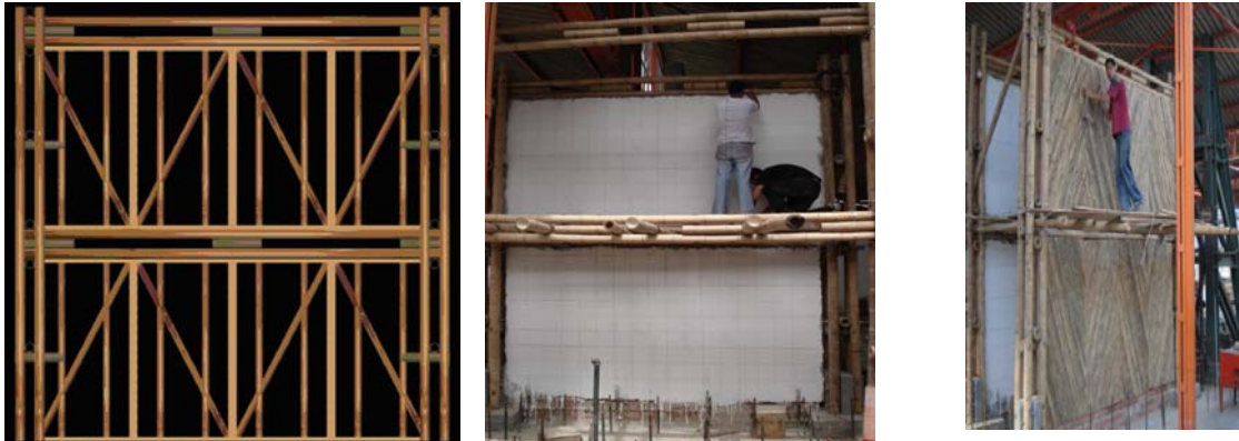
Figure 10. Drawing of guadua frame with the structure of four boards for floor. Frame with boards of bahareque encementado. Frame with board with narrow sheets cover.
